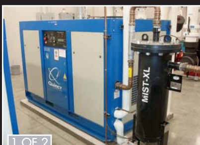
QUINCY MODEL QSI-500 POWER SYNC AIR COMPRESSORS
