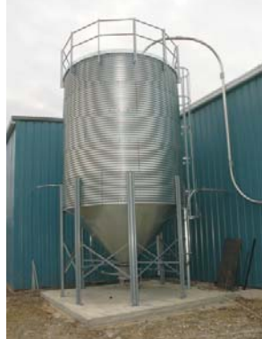
BULK RESIN SILO
